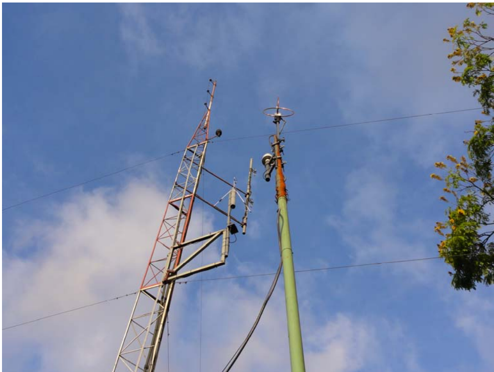
Figure 1 - LMA and LINET antennas installed at Ribeirao Pires site.
