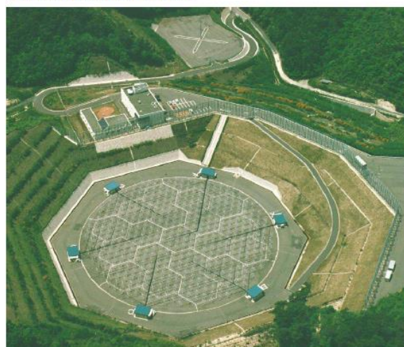
Figure 2: Middle and Upper Atmosphere (MU) radar of the University of Kyoto at Shigaraki, Japan, operating at 46.5 MHz. Constructed 1984.
